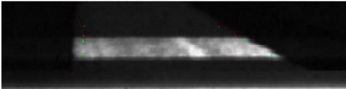
Figure 5: A wide edge line at a motorway with strong wear at the left-hand side towards the traffic.
