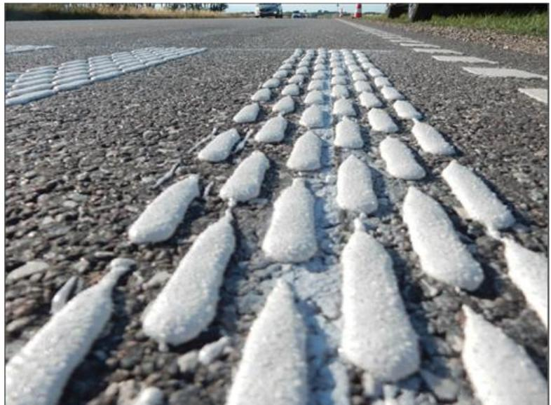
Figure 1: A profiled road marking with directionality of the  $R_L$  and  $Q_d$  values.
